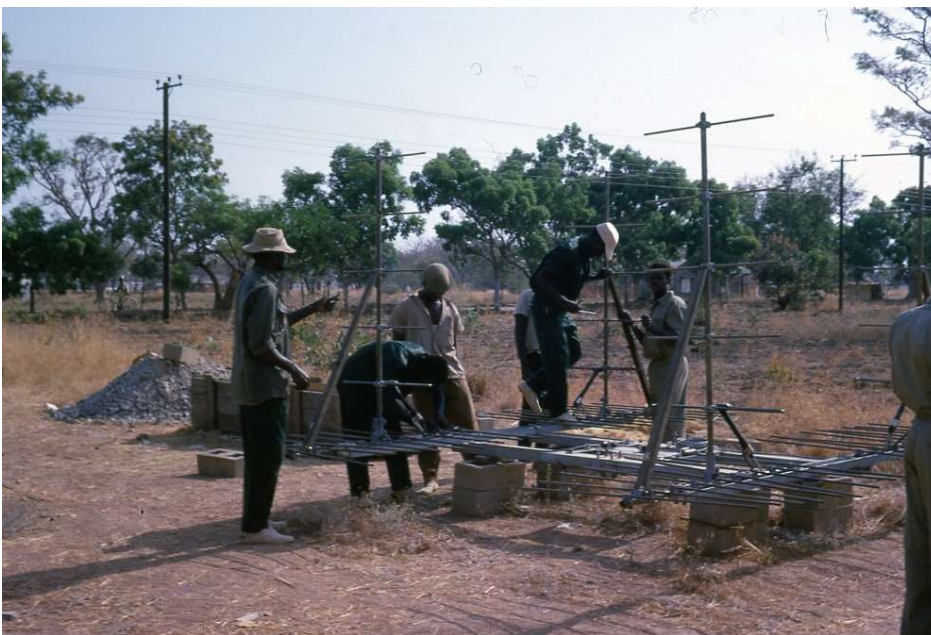
Assembling 4 stack VHF yagi aerial arrays Bauchi, Nigeria 1961
